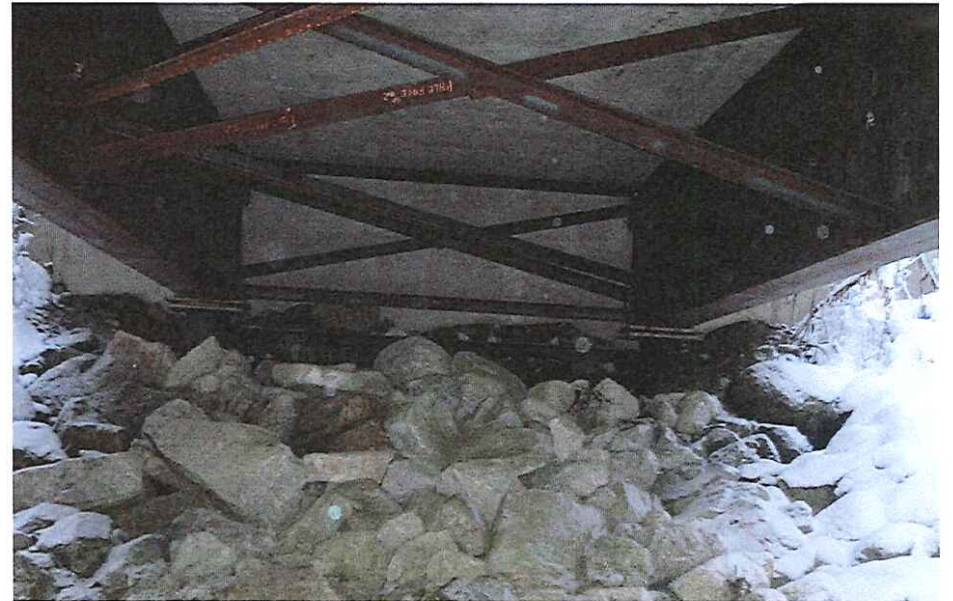
CK-2051 Abutment Left Bank
