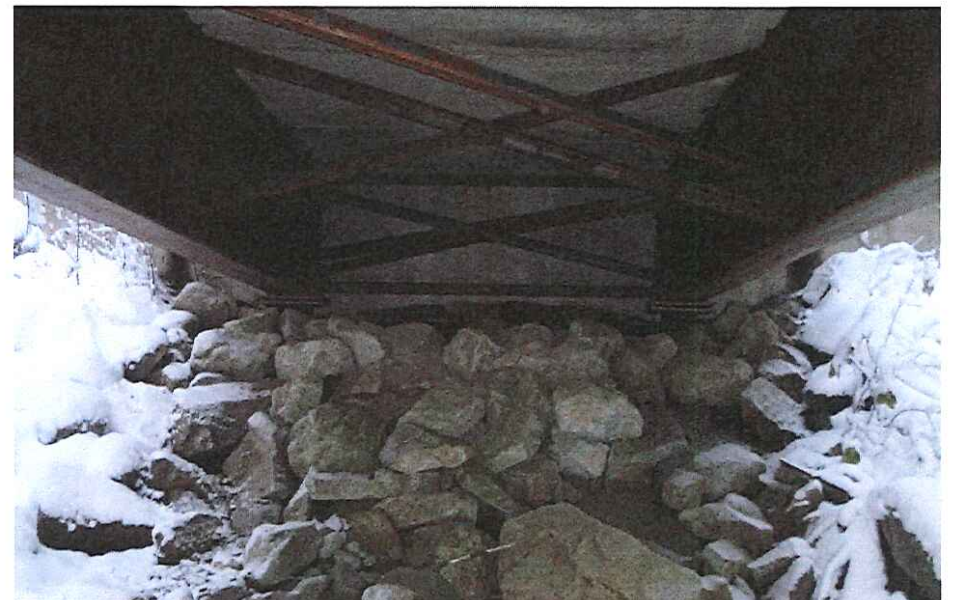
CK-2051 Abutment Right Bank
